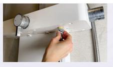
Connect the enclosed 80cm hose to the faucet and the SPASYS body inlet (left)
